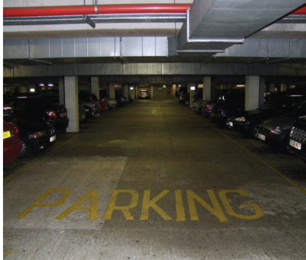
The Lanes aisles before renovation
