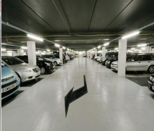
After refurbishment –easier to navigate, brighter for improved safety
