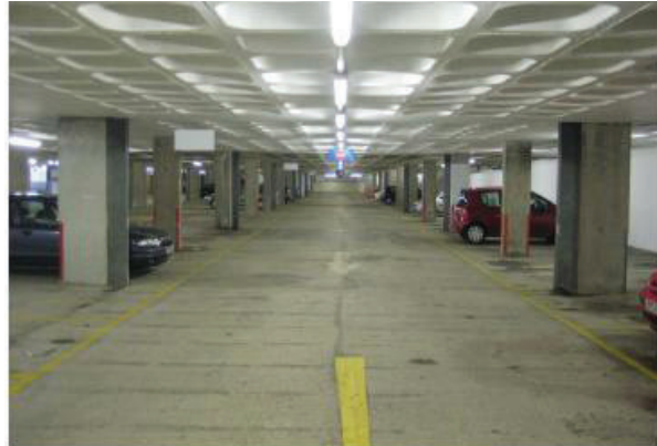
Improved lighting levels, lower energy fittings, surfaces blast washed
